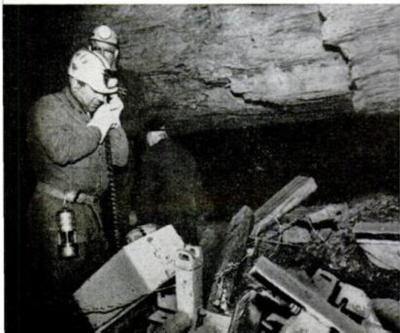
RECOVERY CREW ENCOUNTERED roof timbers, power cables, pieces of primer cord inside mine
